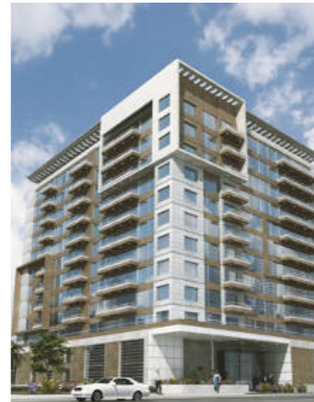
RIGHT: AVENUE RESIDENCE 1
