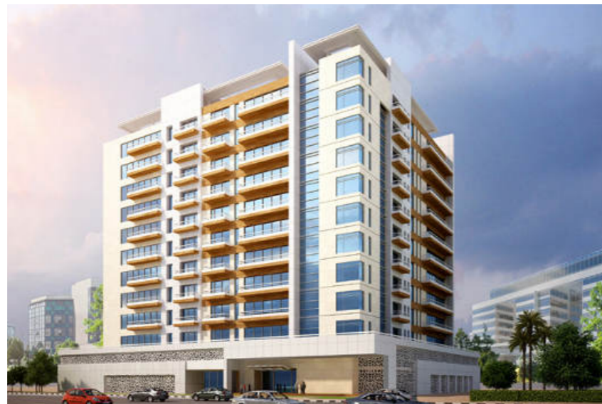
RIGHT: AVENUE RESIDENCE 4
